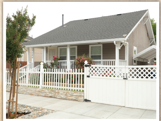
7280 Rosanna Street painting and sensitive renovation
