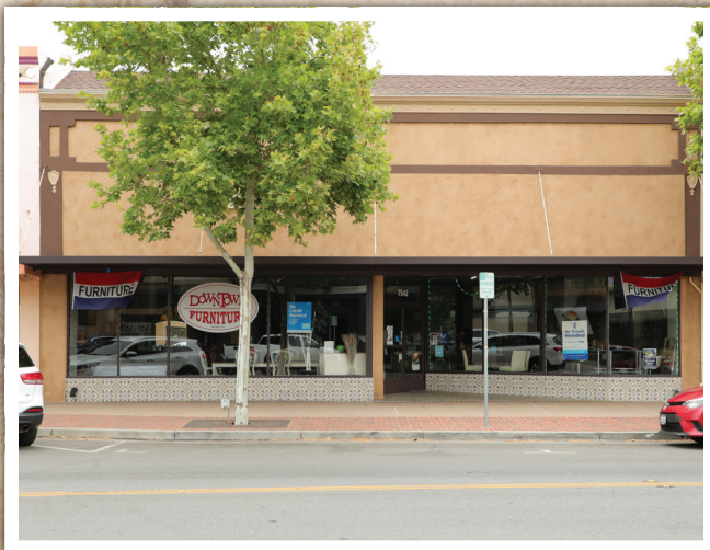
7542 Monterey Road façade painting and tile
